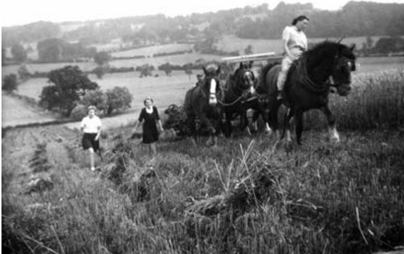
Reaping with a horse-drawn self-binding reaper at Home Farm, Hambleton. Arthur Wild continued to use horses until well into the 1950s, but by this time many farmers had adapted their binders so that they could be drawn by a tractor. Others had been using combine harvesters since before the Second World War (Joan Wild)
