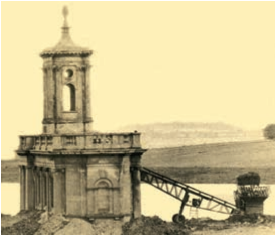
Above: Normanton Church in the process of being saved (Anglian Water)
