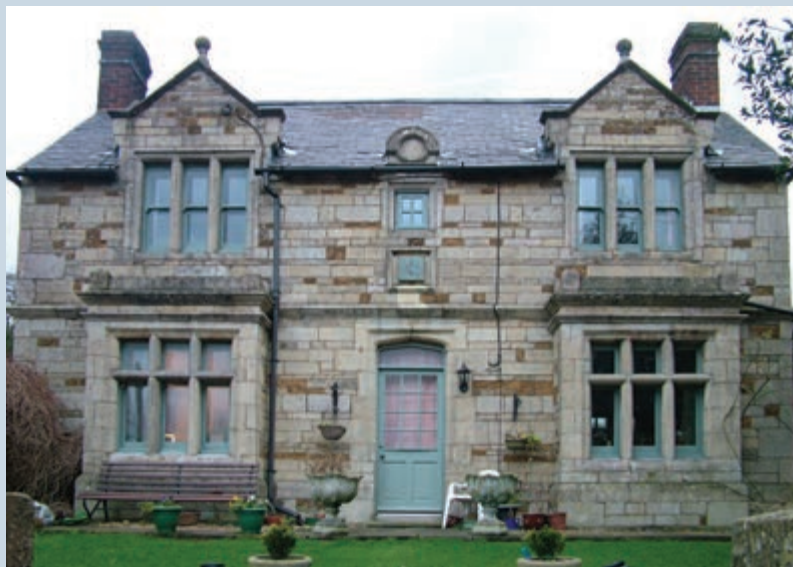
Left: Reclaimed stone and windows from Normanton Hall were used when this house at Knossington, Leicestershire, was built (RO)
