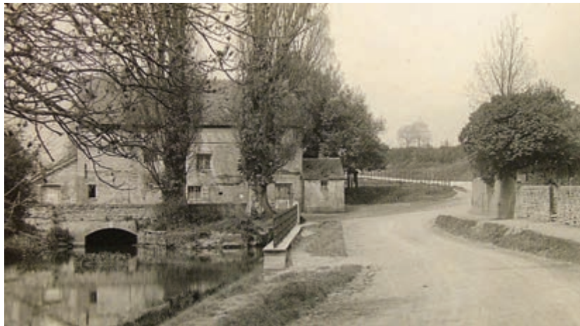
Ryhall Mill in 1925, now demolished (Hart)
